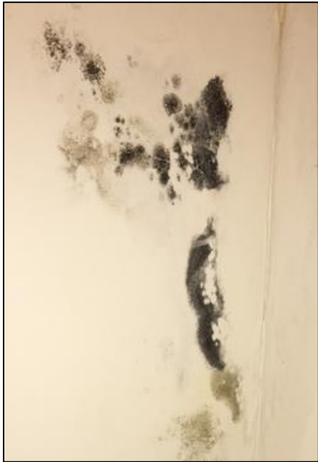
Figure 2: Mold on the wall of a rapid re-housing unit.
